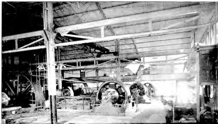
In the Power House of the Electric Railway.
